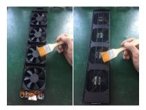
Step 3: Loosen the locking screw to separate the dust screen and fan. Clean the screen and fan by brush.
